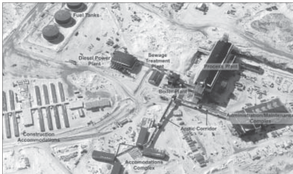
This top down aerial shows the Diavik Diamond Mine infrastructure at the South Camp.
