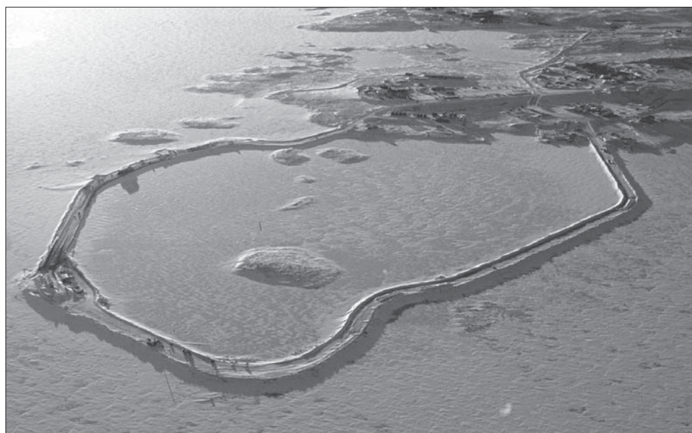
By mid-November, winter's grip had locked Lac de Gras' East Island and the 3.9 kilometre Diavik A154 dike. A month before, the dike embankment was closed in.
