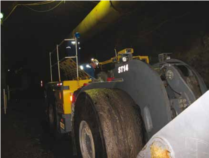
The system, which includes outfitting the scooptram, allows the equipment to be operated from surface and autonomously. Jack Whitford and Martin Champagne of Atlas Copco install the required hardware.
