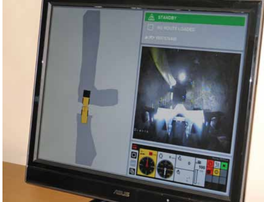
The automated technology's computer hardware displays the scooptram's controls and the machine's location in one of the underground tunnels.
