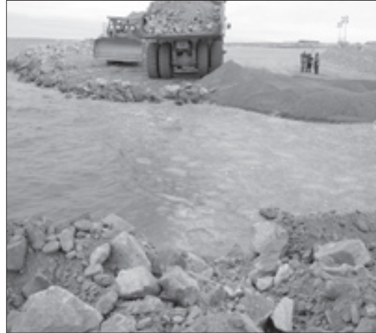
By mid-summer rock placement for Diavik's second dike was well advanced, right, and on October 15 (above) workers closed the remaining gap.
