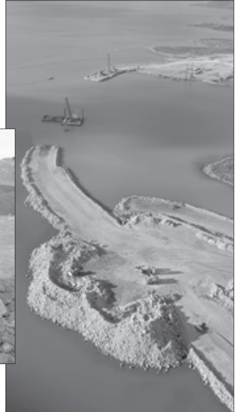
By mid-summer rock placement for Diavik's second dike was well advanced, right, and on October 15 (above) workers closed the remaining gap.
