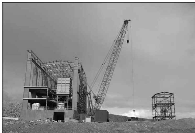
Diavik's new crusher plant under construction.
